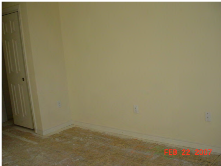
Wall Partition in Condominium 2009 Bedroom, Second Floor
